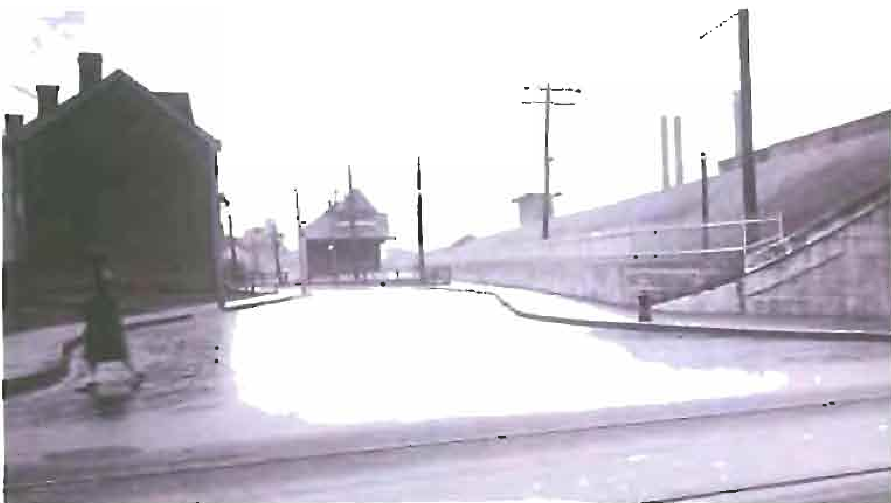
December 1930. The completed embankment/underpass at De Grassi. City of Toronto Archives, Series 372, SubSeries 79, Item 601
